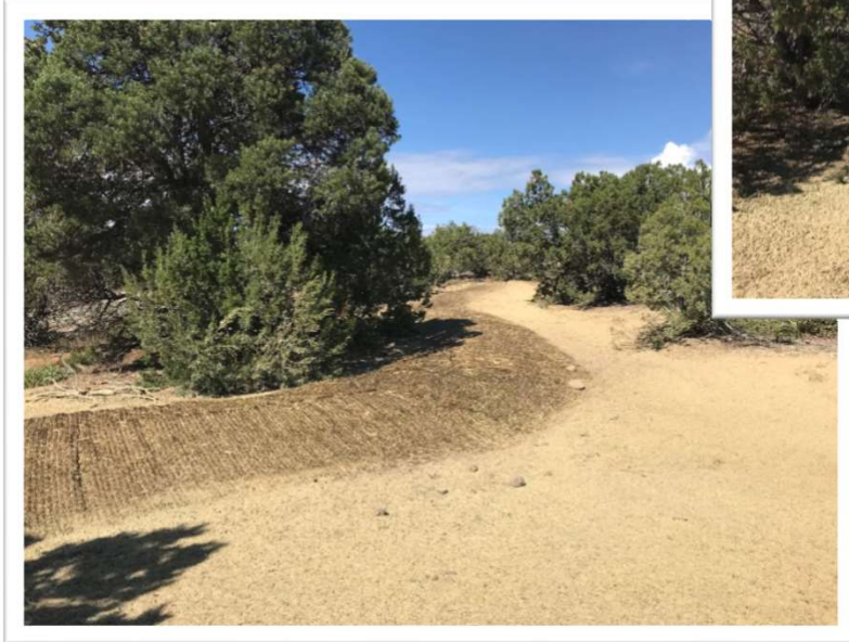
Diversion berm, modified retention berm, and new retention berm with rock apron
