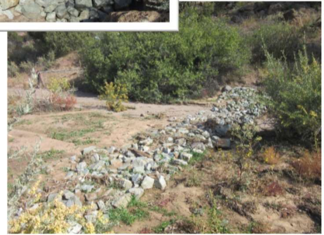
Three rock check dams with armored pools and a one rock check dam
