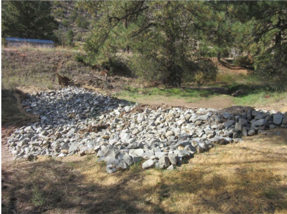
Rock check dam with apron
