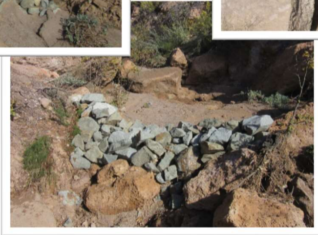
Three rock check dams with armored pools and a one rock check dam
