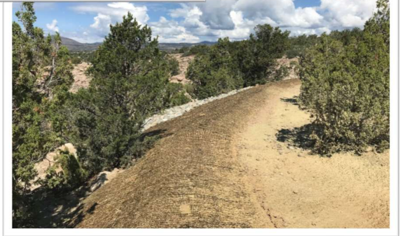
Diversion berm, modified retention berm, and new retention berm with rock apron
